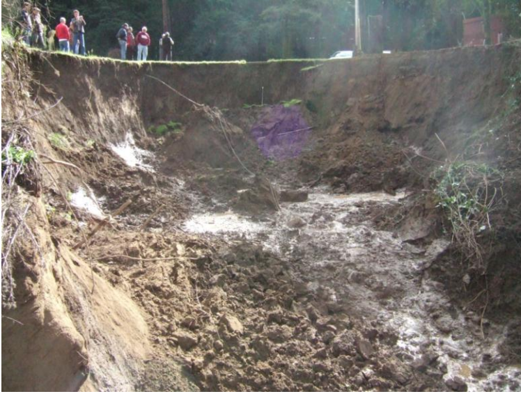
Above Left: February 2008, Before Restoration
